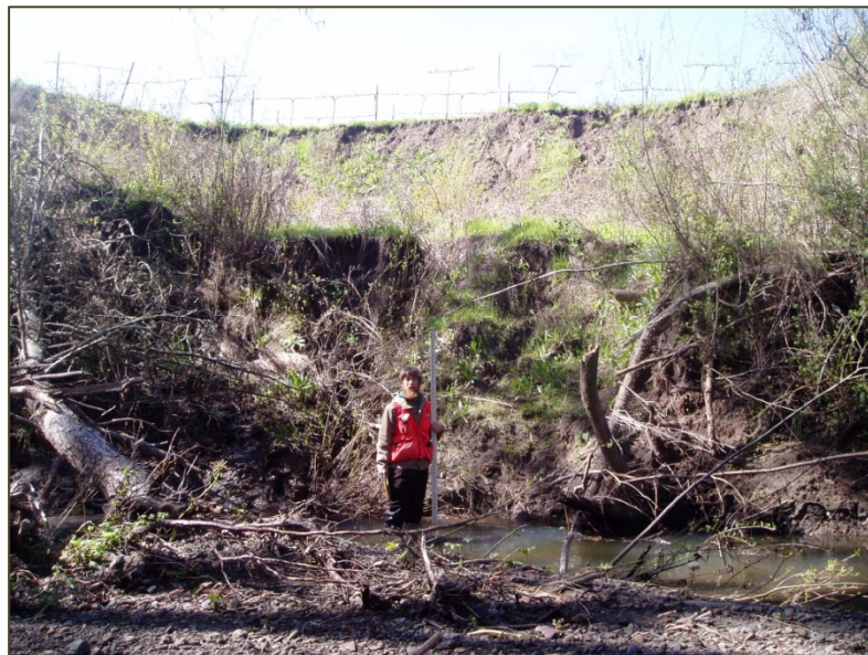
Bank Collapse/Erosion. Photo courtesy of Matt O'Connor.
