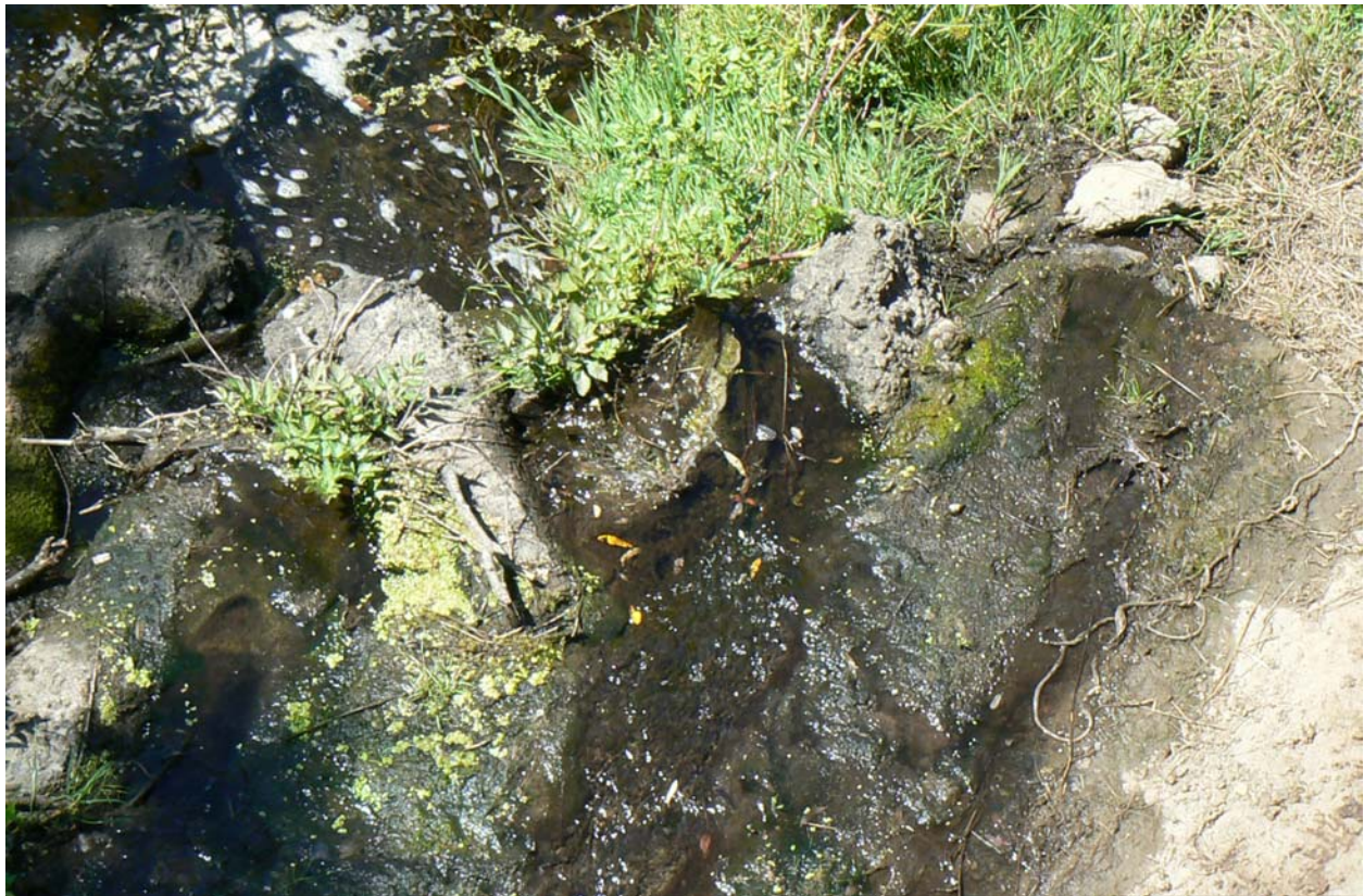
August 12, 2011 trickle of streamflow over the culvert at Station EBC-30
