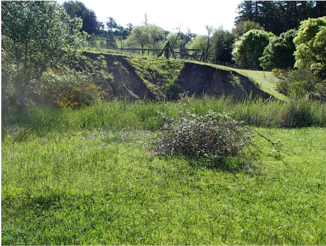
Photo 3. View looking across the stream at Site B bank erosion (March 2015)
