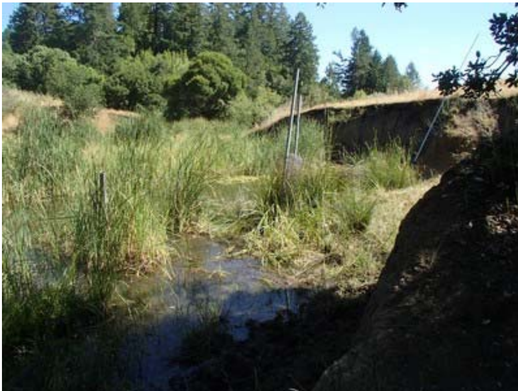
Photo 2. View looking downstream at Site A bank erosion (June 2016)
