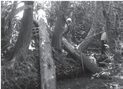
Installation of large woody debris for fish habitat.
