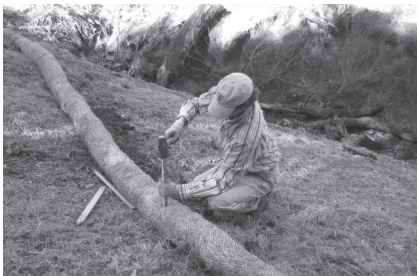
Erosion control installation. Little Black Mountain, Austin Creek
