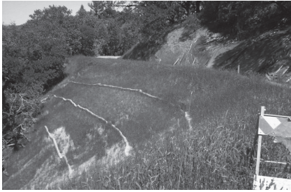
Pena Creek Watershed. Slide stabilization.
